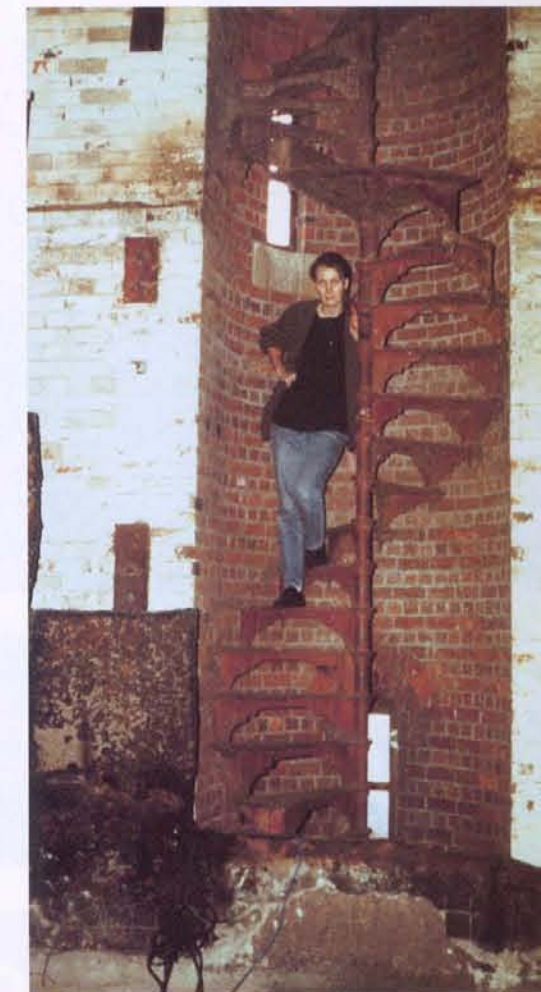
When Godalming-based architect Elspeth Beard bought Munstead Water Tower for £121,000 at auction in October 1998 she became the proud owner of a Grade II listed building that had stood derelict for nearly 20 years and came complete with a 2ft layer of pigeon droppings
